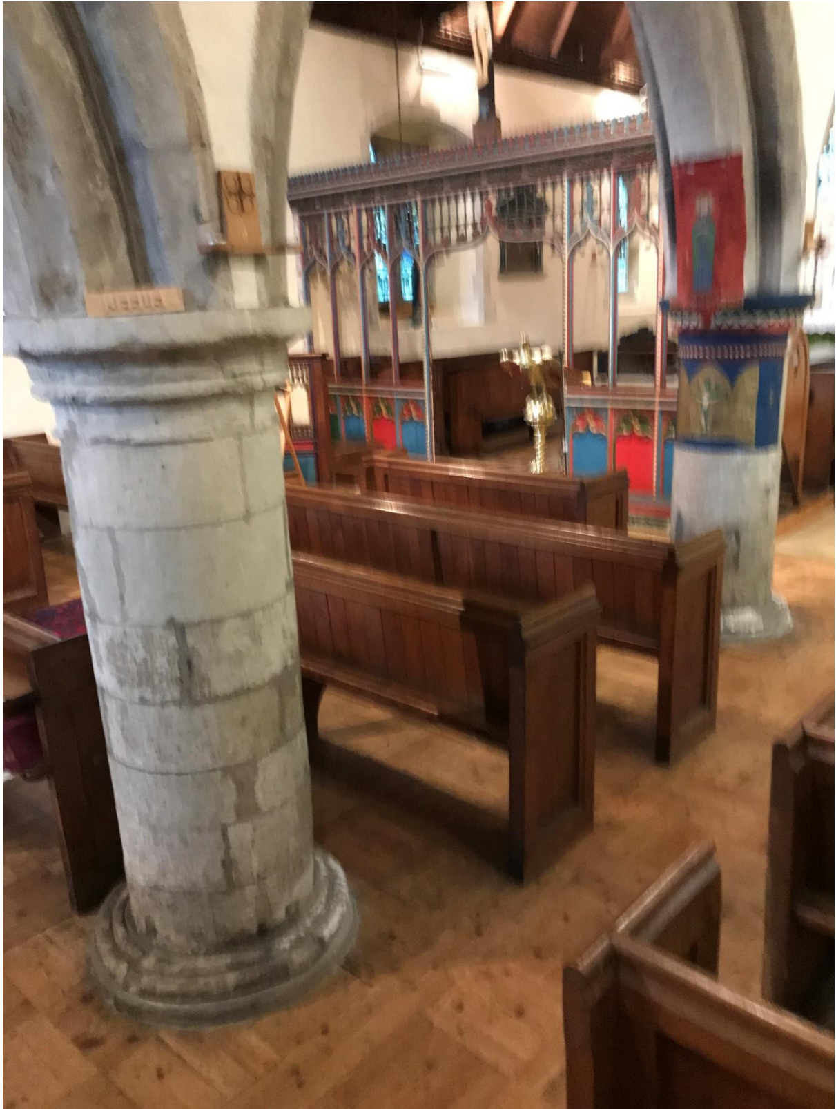
South Aisle pillars from south chapel
